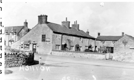
One of many stand pipes located on Crown Corner. Look just above the "TO" of ASHTON
